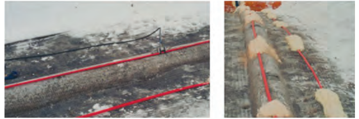
Two fiber sensor arrays deployed with the Ventometer.
